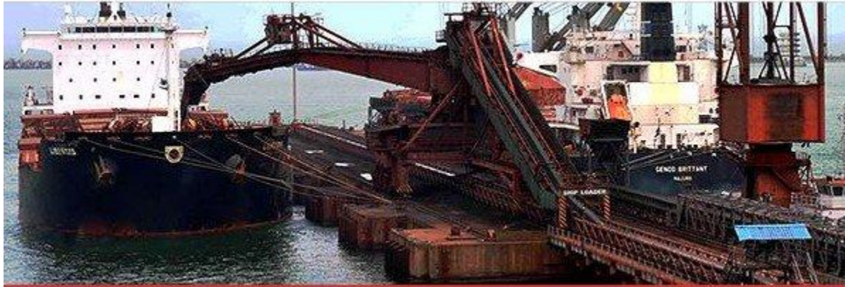
Pic : The fully mechanized ore handling plant of VPT upgraded by ESSAR Vizag Terminals Ltd on PPP mode.jpg
